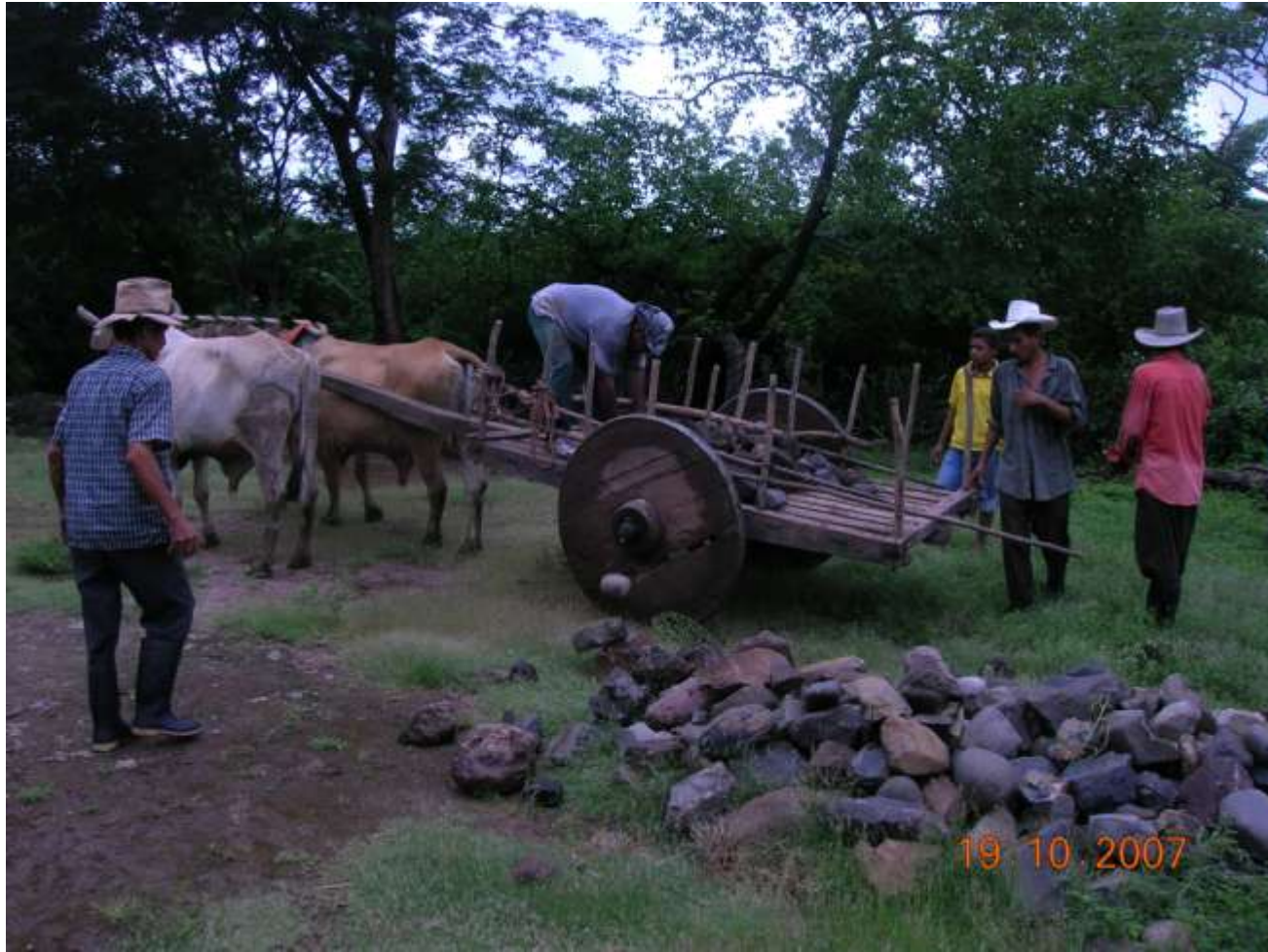
Foundation rocks and concrete sand is delivered to the kitchen site
